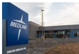
Medline Renewal Building -Photo Courtesy: Tim Park
